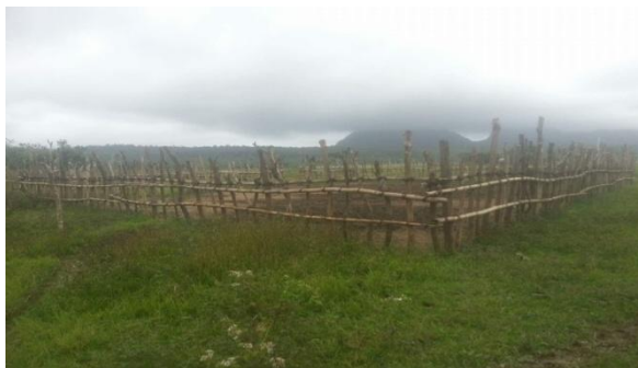
Figure 2. Construction of Balinese cattle cage in District Tutuala
